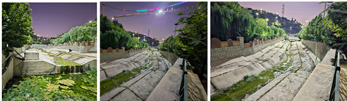
Figure 6. Channelized bed in Nahj al-Balaghah Park
